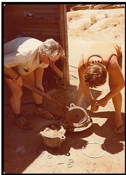
Panning for gold and melting and pouring the gold at Sothern Cross – Marvel Loch
